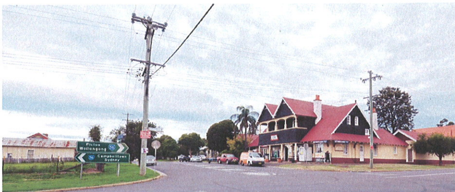
Village centre: Menangle Store, Barn, Hall, and Cottage, Corner Station St. and Woodbridge Rd's
